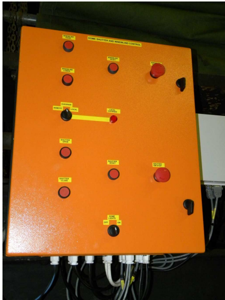
This cabinet also contains all the drive electronics.
